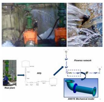
tripping or valve closure. Generally speaking, Flownex is a Computational Fluid Dynamics (CFD) system simulation software that solves equations for conservation of mass, energy, linear and angular momentum. Its fundamental approach is based on a thermal-fluid network of 1D
